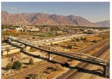
The structure is intended to move as much as 18 inches and in every direction all the time: left to right, backwards and forwards, up and down.
