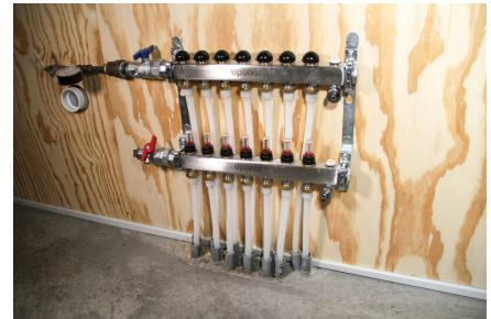
Besides offering a higher flow velocity compared to CPVC or copper, a PEX system holds a smaller volume of water than the same-sized system using either of these materials in the same pipe diameters.
